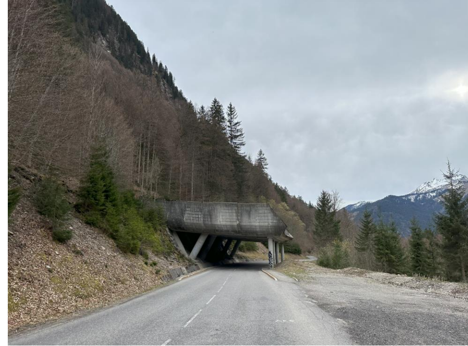
Avalanche protection on the roads, Montriond
